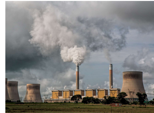
Point source capture (PSC)
