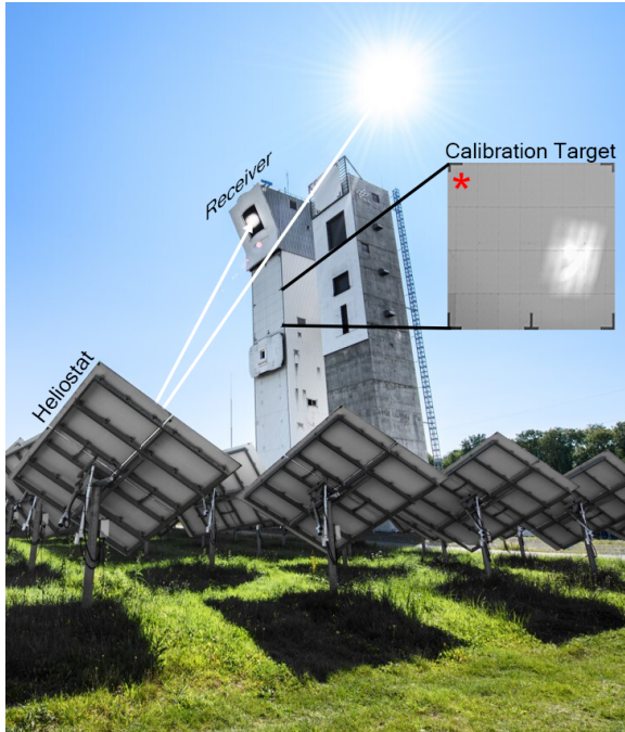
Fig. 1: Image of the two solar towers in Jülich. The heliostats, shown from behind, are focusing sunlight on the receiver surface of the left tower. Located below the receiver is the calibration target. The inset shows a focal spot image as it is taken during calibration.
