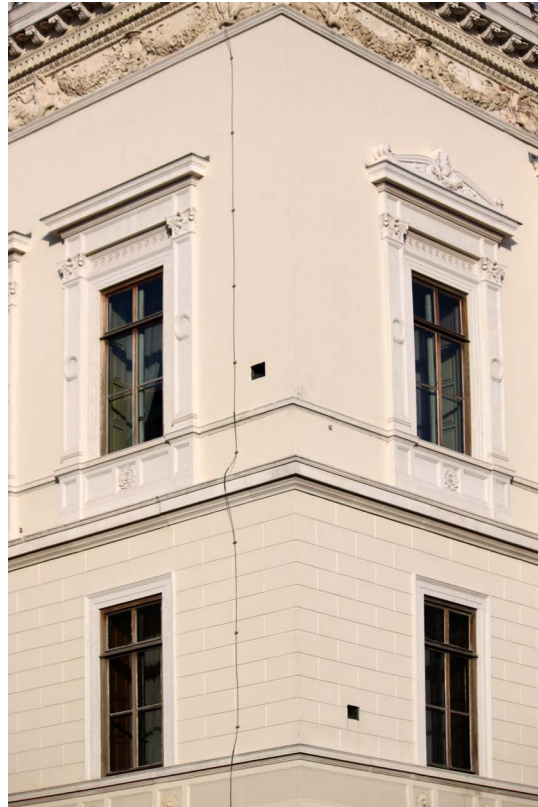
FIGURE 3.44: Revoltella palace from the outside. Two black rect- angular holes in the wall, which house the lenses of two dark cham- bers, are visible from Piazza Venezia.
