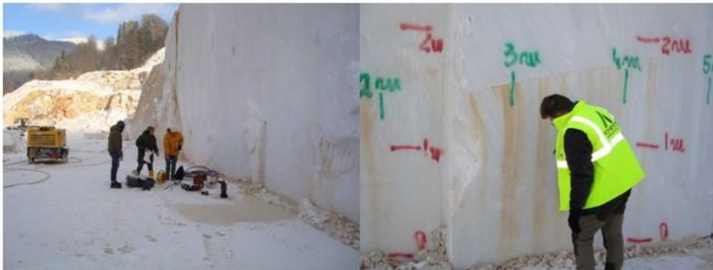
Figure 17. Main wall of the block marble west-facing for televiwer and scanline measurements
