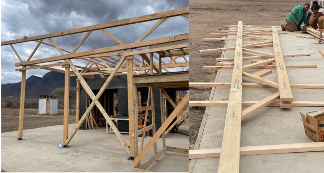
Figure 2: Permanent Structure Roof Truss
