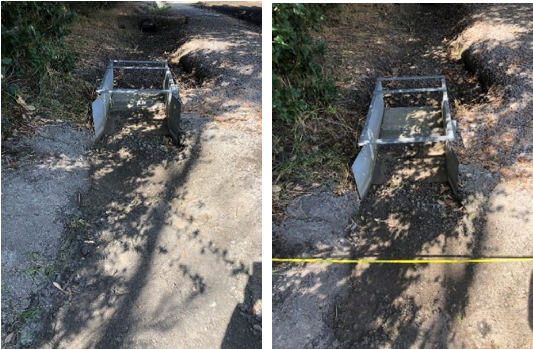
Figure 17. Concrete channel testing location
