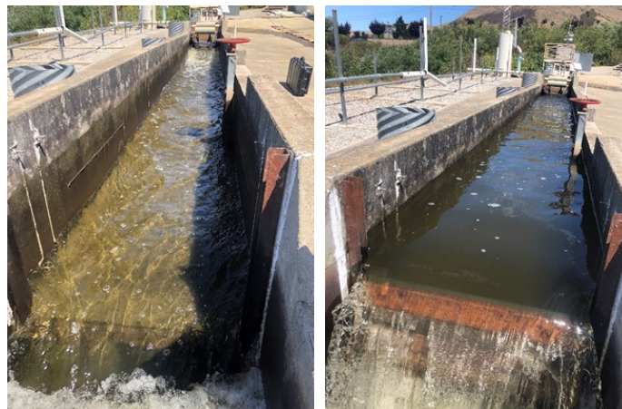
Figure 24. Rectangular channel without flashboards (left) and with four flashboards (right)
