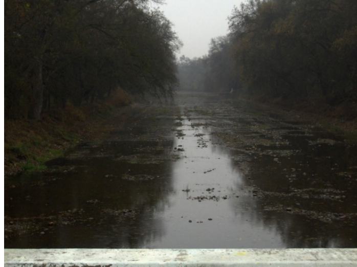
Figure 42. An example of a cross section made of rocks in a large channel; the rocks look small but can be seen in patches out of the shallow water
