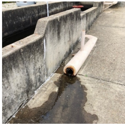
Figure 23. Gate leak
