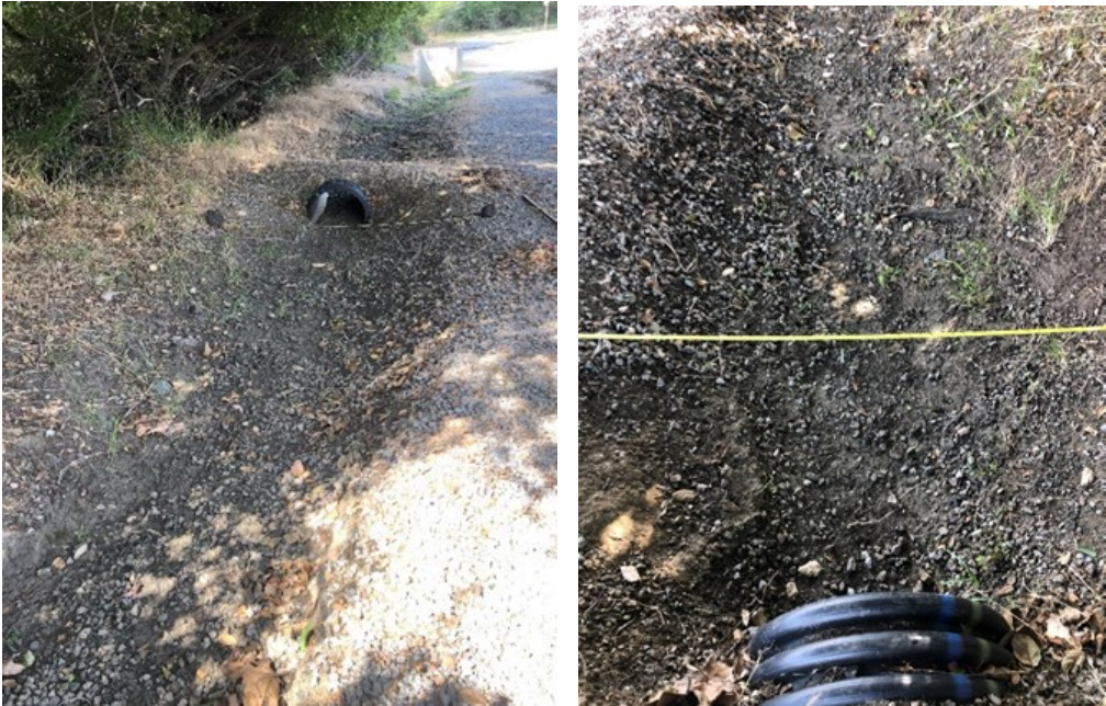
Figure 19. Earthen channel testing location
