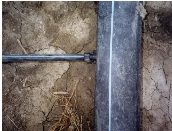
Figure 1. Manifold connection with "quick release" fitting directly connecting PE oval hose manifold to the tape.
