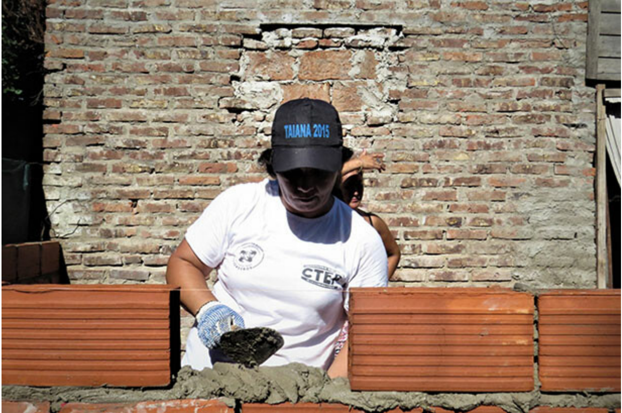
Figure 3. Silvia working on renovation of a cooperative member's house.
