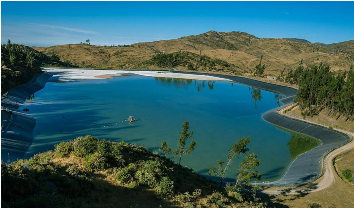
Figure 26. Gold tailings storage facility where the entire reservoir area is lined with a multilayer geosynthetics system.
