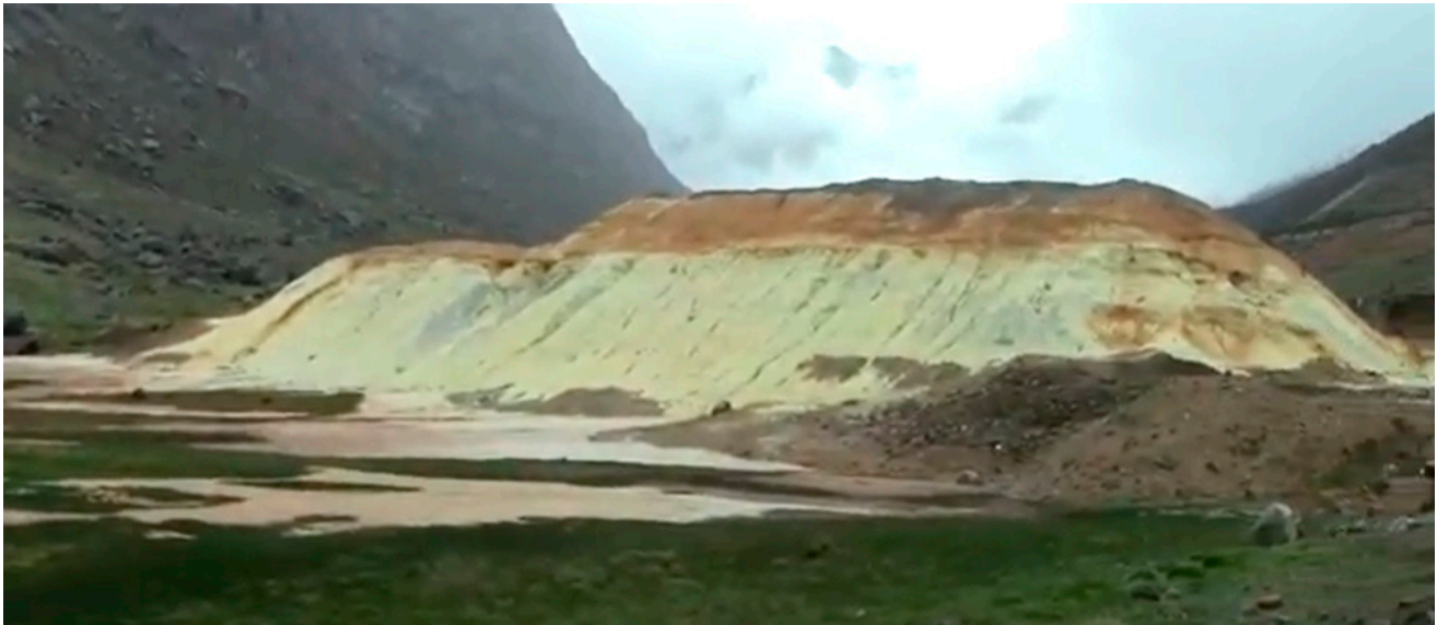
Figure 23. An abandoned tailings storage facility in the Andes mountains showing oxidation of mine tailings.
