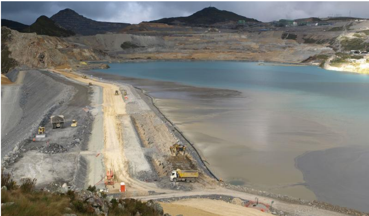
Figure 13. View of copper tailings storage facility located close to concentrator plant, showing conventional use of tailings.
