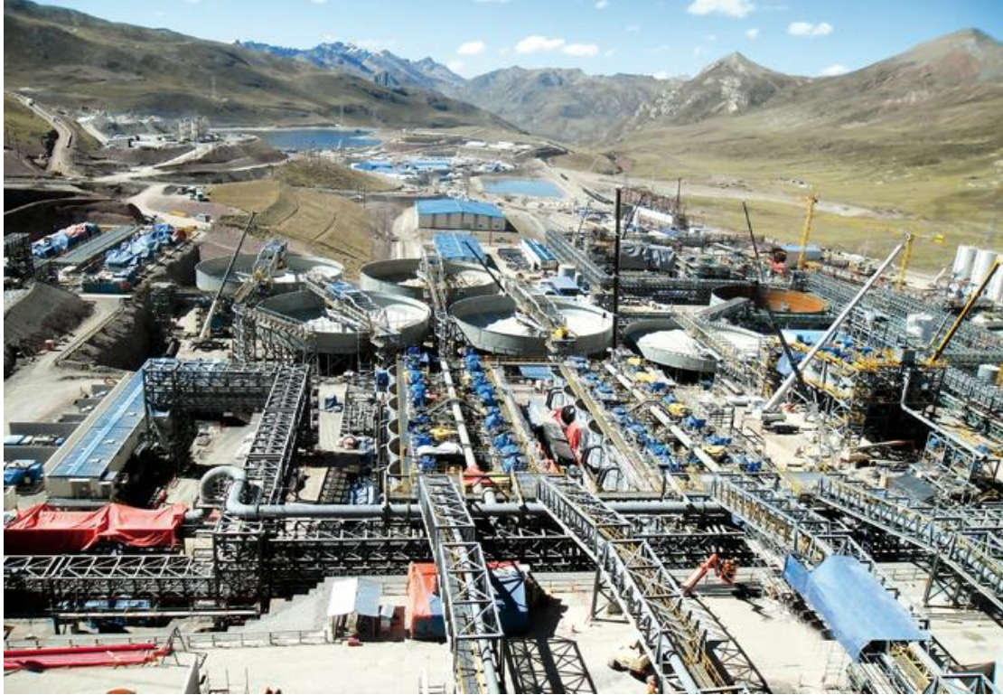
Figure 12. Typical view of sulphide copper concentrator plant showing flotation cells, tailings thickener, and concentrate thickener.
