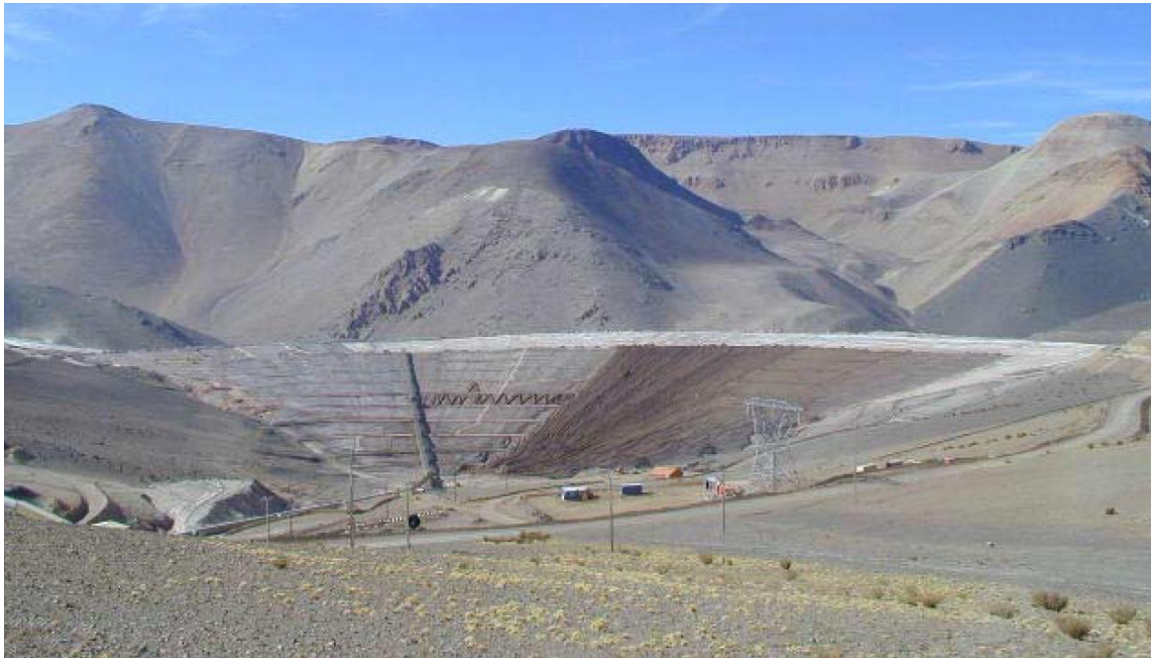
Figure 19. Typical view of gold tailings storage facility showing filtered tailings technology with dry stacking at a mine in the Andes mountains.
