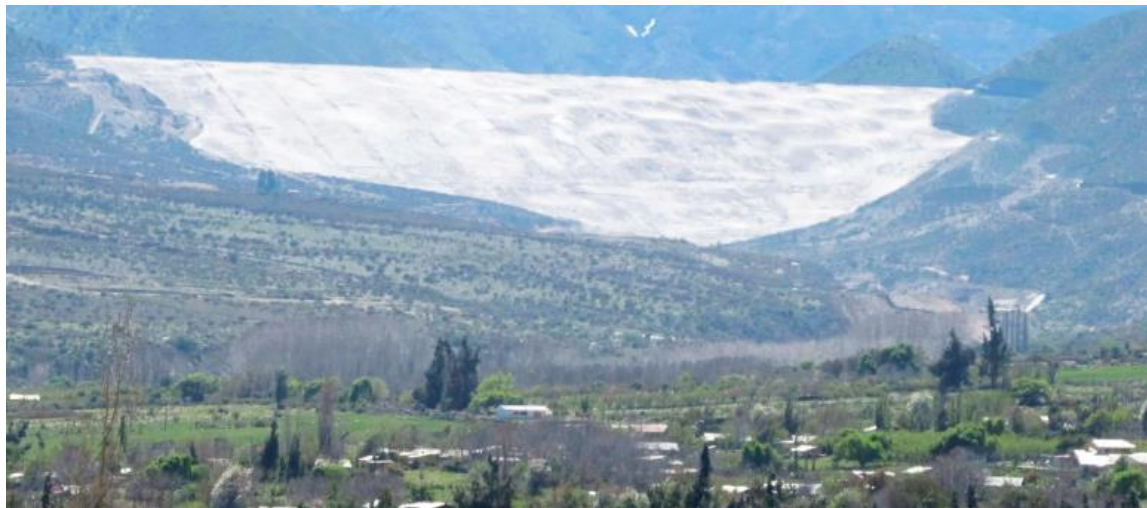
Figure 8. Example of mine tailings disposal in a valley: Cycloned Tailings Sand Dam, Chile, 200 m in height.
