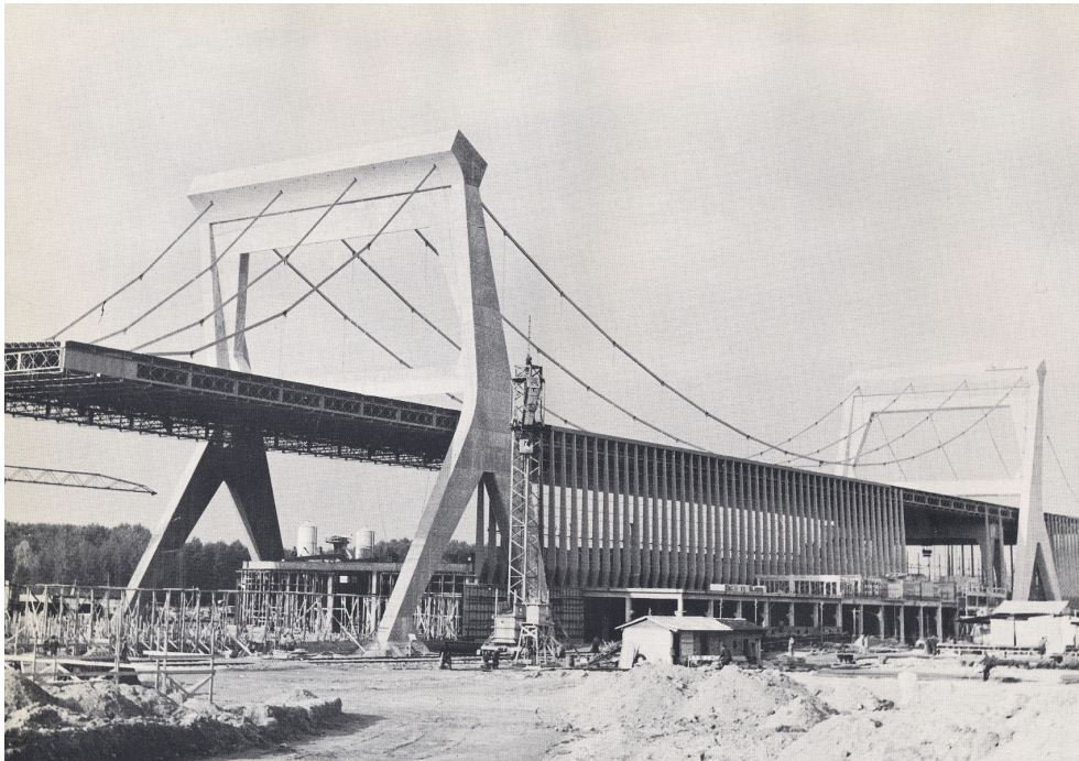
Figure 7. The Burgo Paper Mill in construction [MAXXI]
