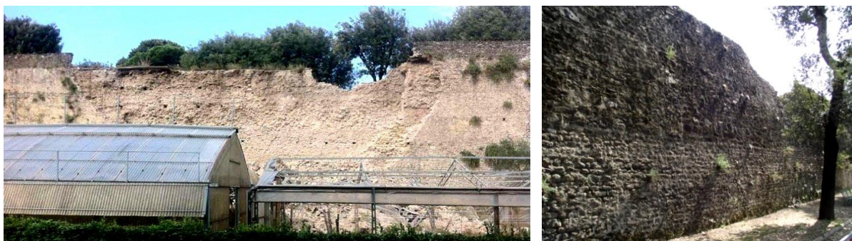
Figure 1: Collapse of the city walls of Pistoia (September 19, 2011). On the left: the failure seen from the outer side; on the right: the failure seen from the city centre.
