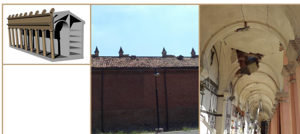
Figure 6: Monumental cemetery of Concordia Sulla Secchia -Tipping over of the projecting elements away. In this case the projecting elements are collapsed inside the structures
