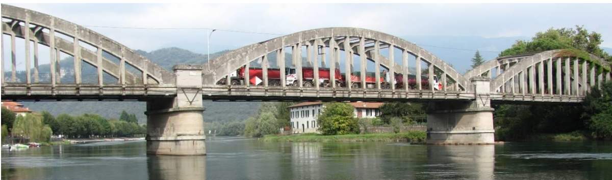
Figure 7: Trucks used during the load test of Span 02.
