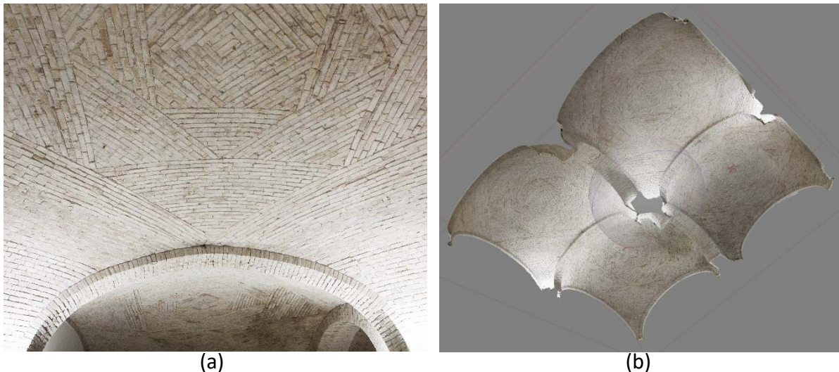
Figure 1. A typical lowered sail vault in Cagliari (a); geometry obtained by laser scanner survey (b).
