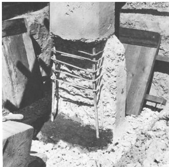
Figure 3 : Repair of footing – 1927 [3]
