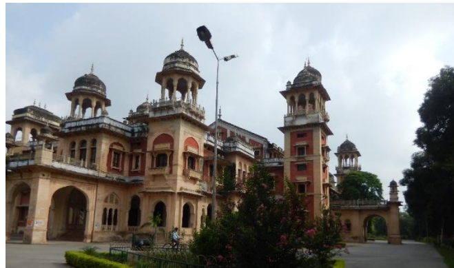
Figure 1: Senate Hall Building, Allahabad university
