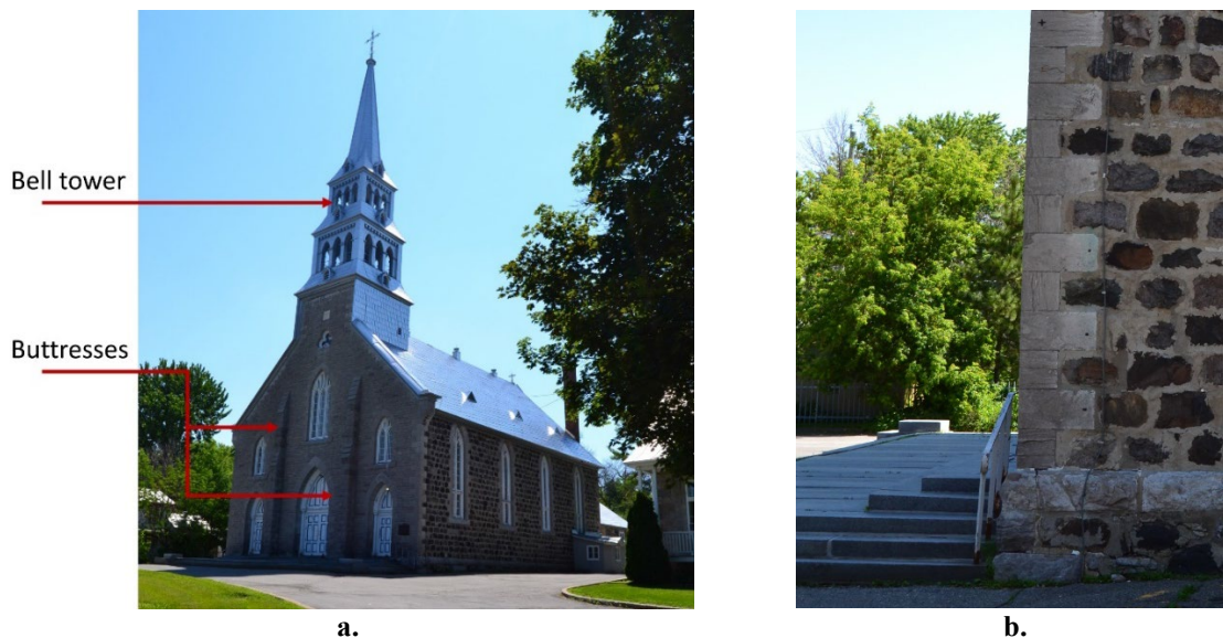
Figure 6 The exterior of the church: a. The principal elevation; b. The detail of interconnection between walls.
