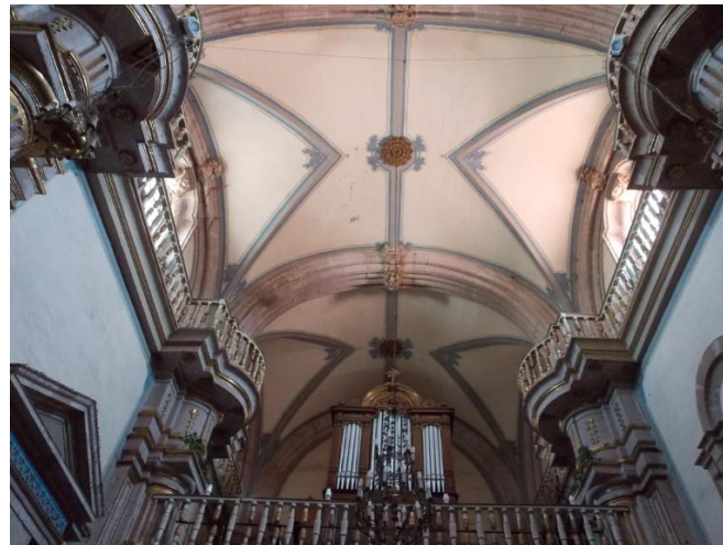
Figure 4: Nave chorus and lunette vaults stiffened with rib arches
