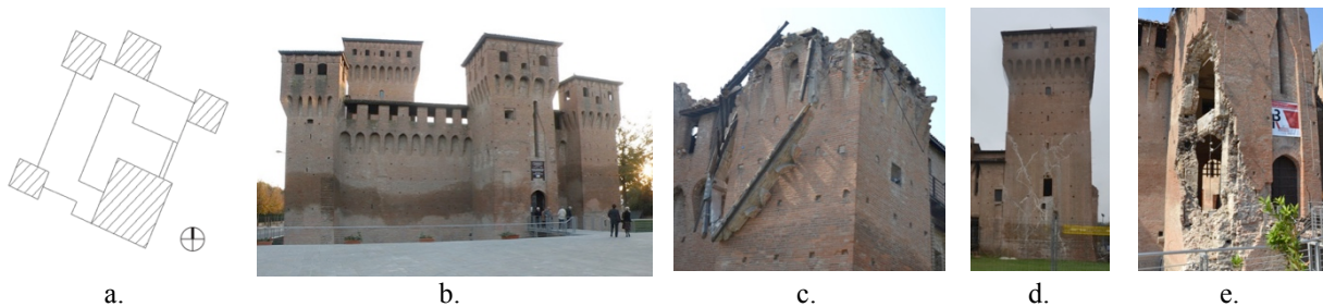
Figure 1: Schematic floor plan (a) and general view (b); examples of collapse mechanisms exhibited by the fortress: collapse of a minor tower's roof (c), damage pattern in the Mastio (d) and collapse in the north tower (e)
