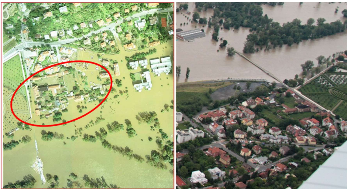
Figure 1: Left: unprotected historic Troja district (Prague, Czech Republic) during flood in the year 2002; right: the same area protected with a combined permanent and temporary wall during flood in the year 2013.
