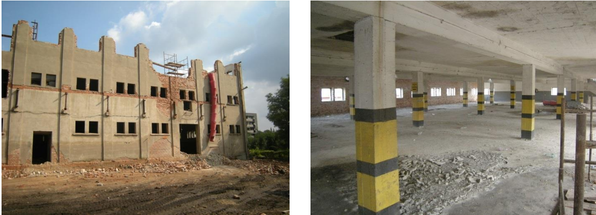
Figure 10: View of warehouse after partial demolition and the rib floor structure in a ground floor (1950)
