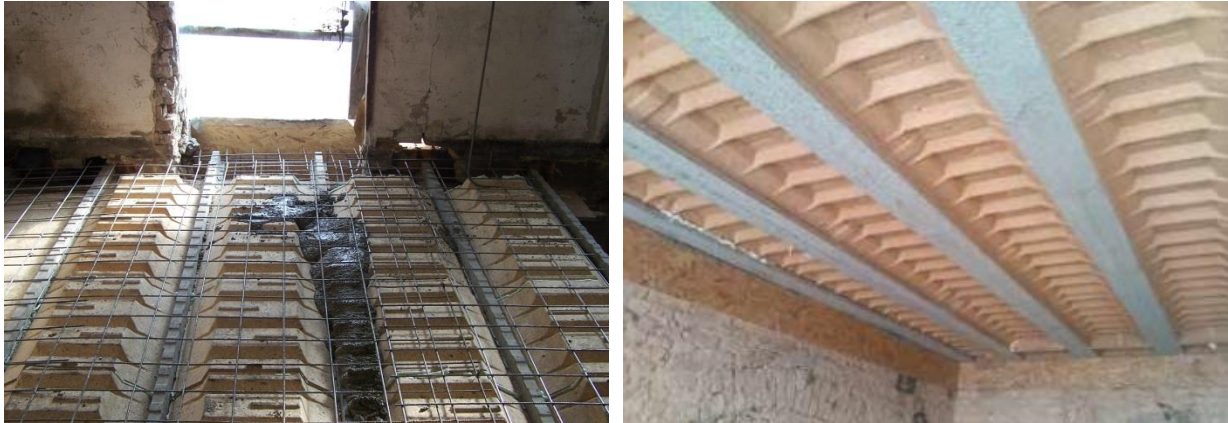
Figure 16: View of the RECTOLIGHT concrete floor
