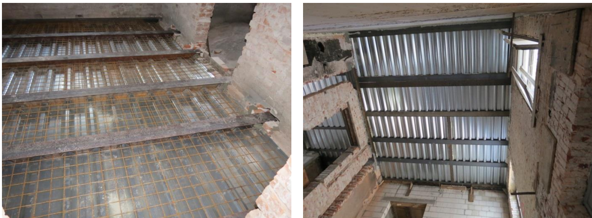
Figure 17: View of the composite floor
