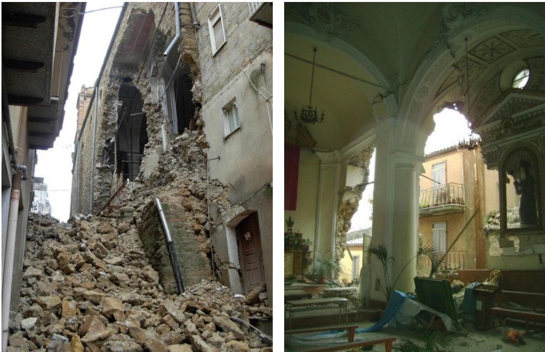
Figure 1: Pictures of the collapse from the outside and inside the church
