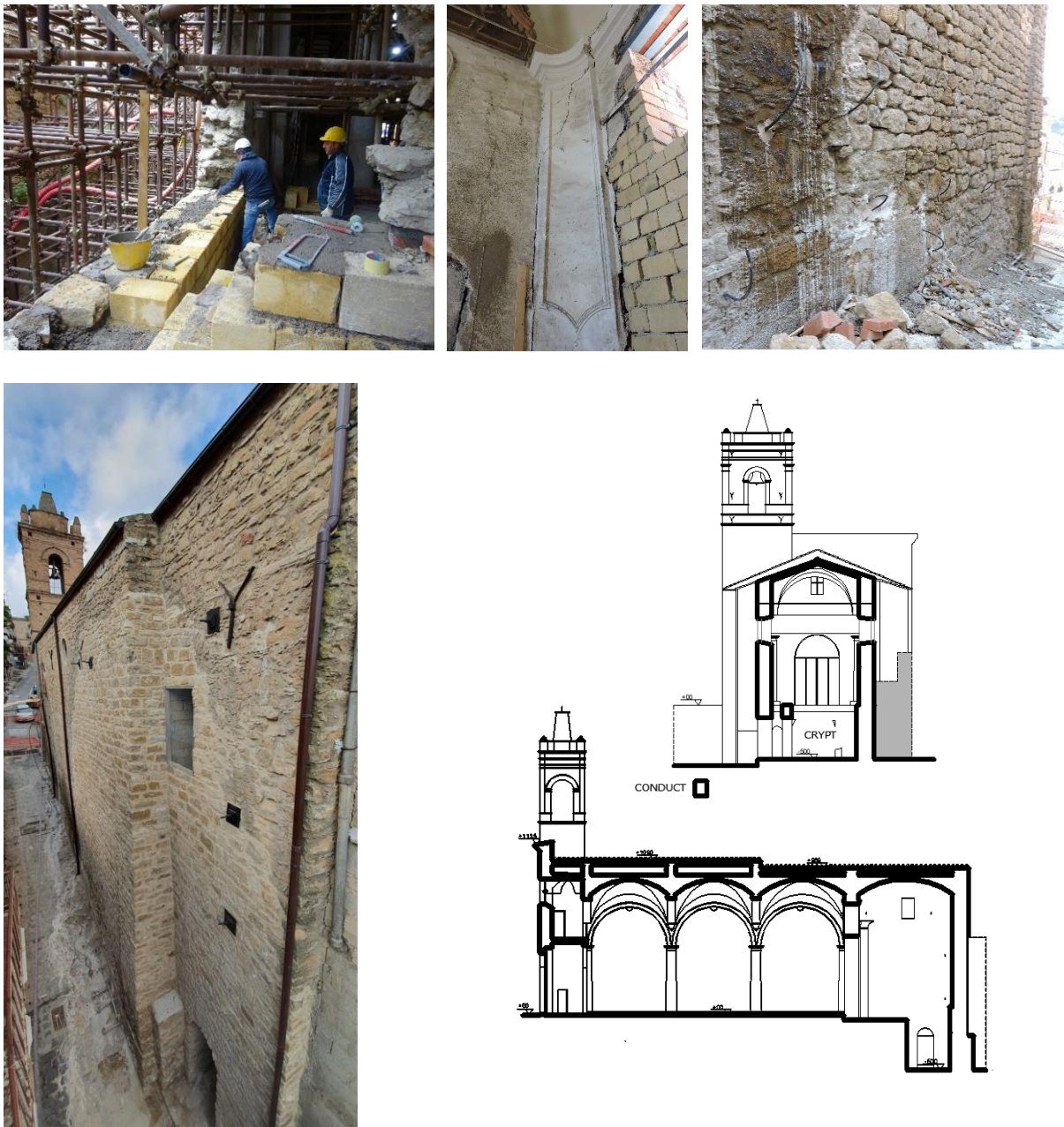
Figure 9: Photographs of the reconstructed wall and drawings of the church with the found underground room
