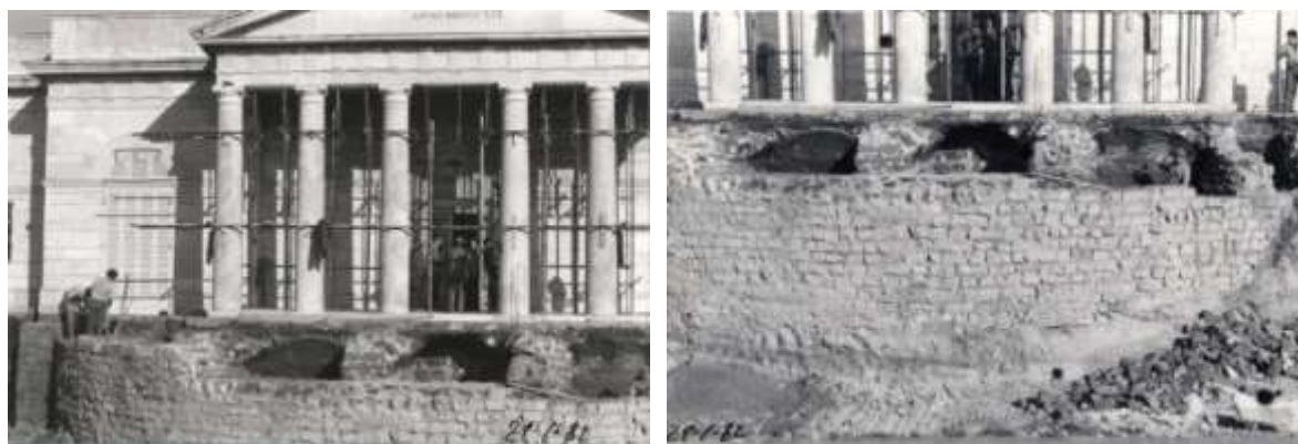
Figure 4: Works for the realization of the Auditorium in 1982.
