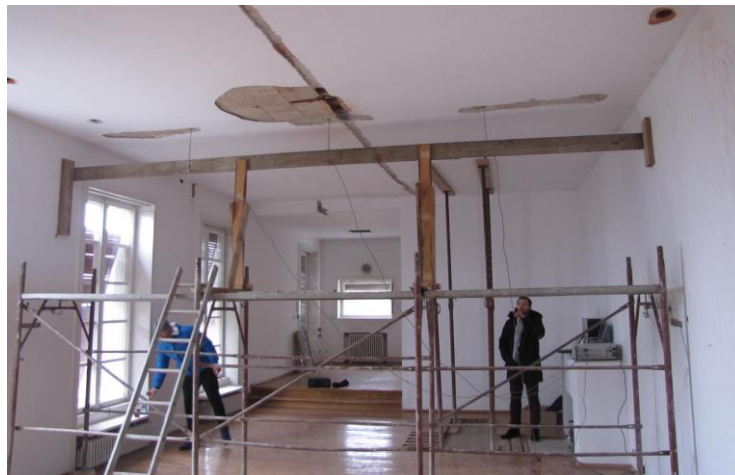
Figure 9: Slab Deflection measurement with displacement transducers
