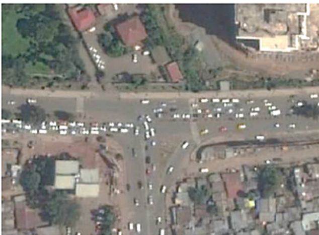
Figure 1. Road Corridor "before" Improvement (Source: [9]).
