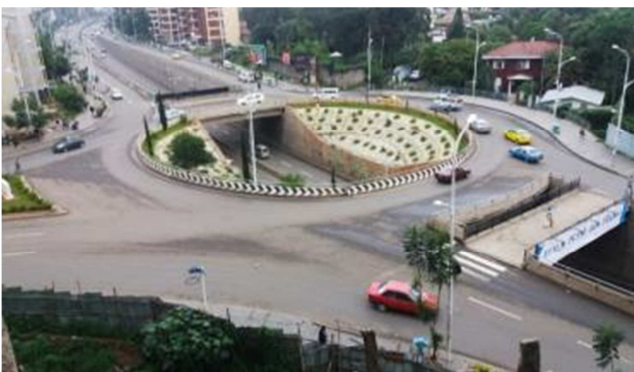
Figure 2. Road Corridor "after" Improvement. Source: Photo Taken August 8/2017.
