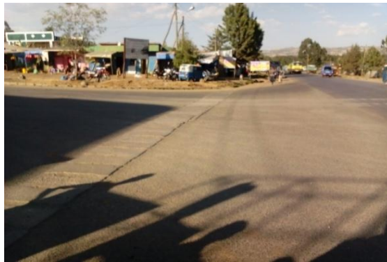
Figure 3.4: Gabriel Existing Road Condition
