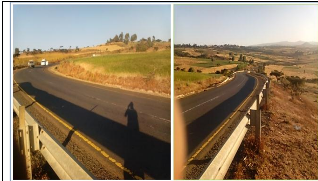
Figure 3.10: Minini Existing Road Condition.
