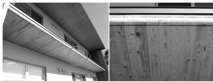
Figure 2. Deformation of CLT exposed to outdoor climate (Eaves of CLT flat roof).
