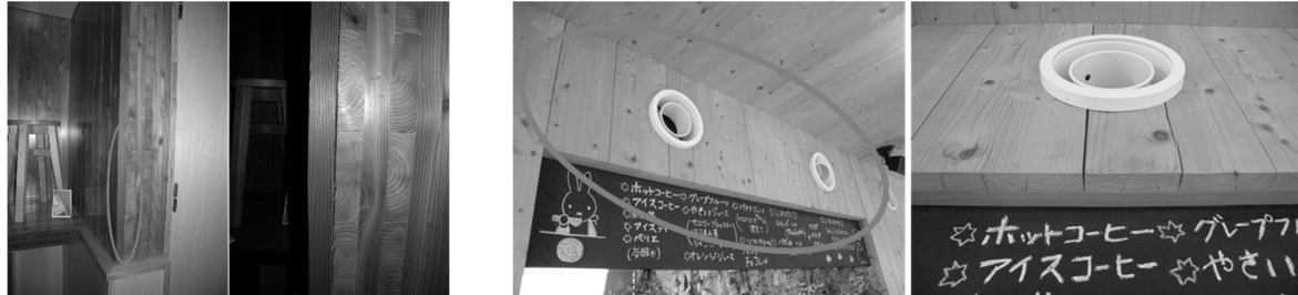
(a) Delamination of the surface lamination. (b) Check and shake of the surface lamination.
