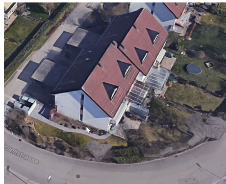
Figure 2. Aerial view of the façade from West.
