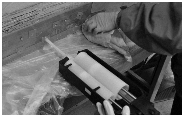
Figure 4. Resin filling work.
