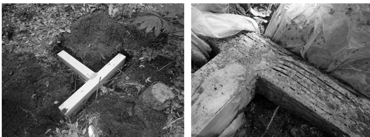
Figure 5. Soil exposure due to feeding damage caused by termites.
