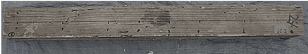
Figure 2. Timber filled with resin.
