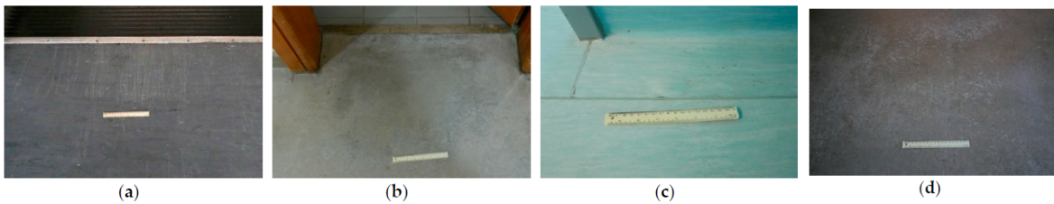
Figure 2. Anomalies: (a) scratches; (b) wear; (c) brightness changes; (d) brightness changes on a linoleum flooring due to inadequate maintenance.
