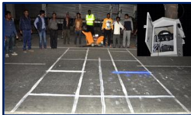
Figure 7. Installation of Loops under Road Pavement
