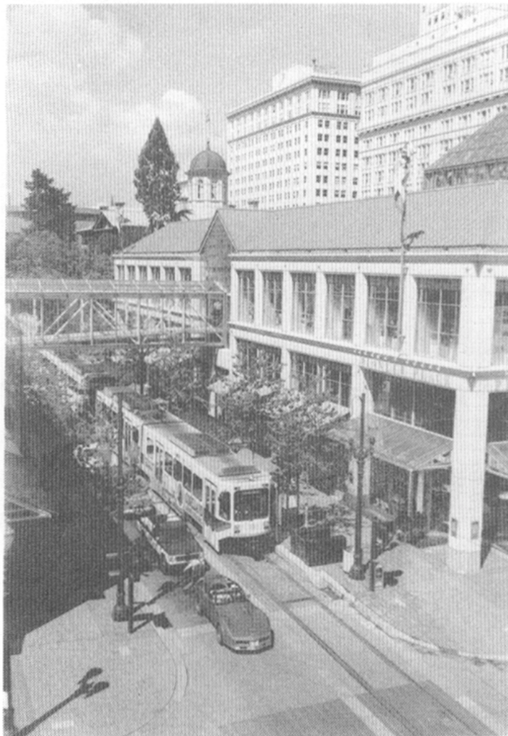
Figure 29. Pioneer Place Light Rail Station
