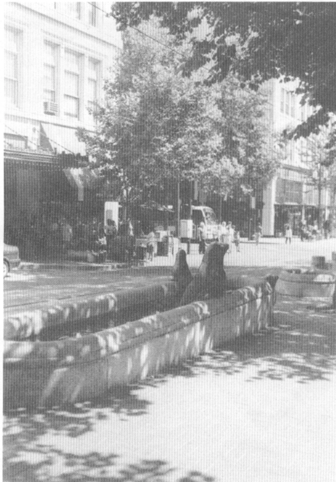
Figure 28. Artwork and Brick Sidewalks Along Morrison Street Light Rail
