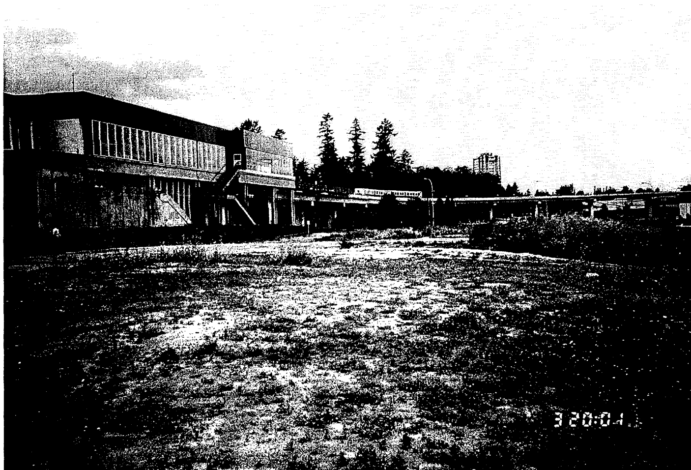
Figure 34. King George Station
