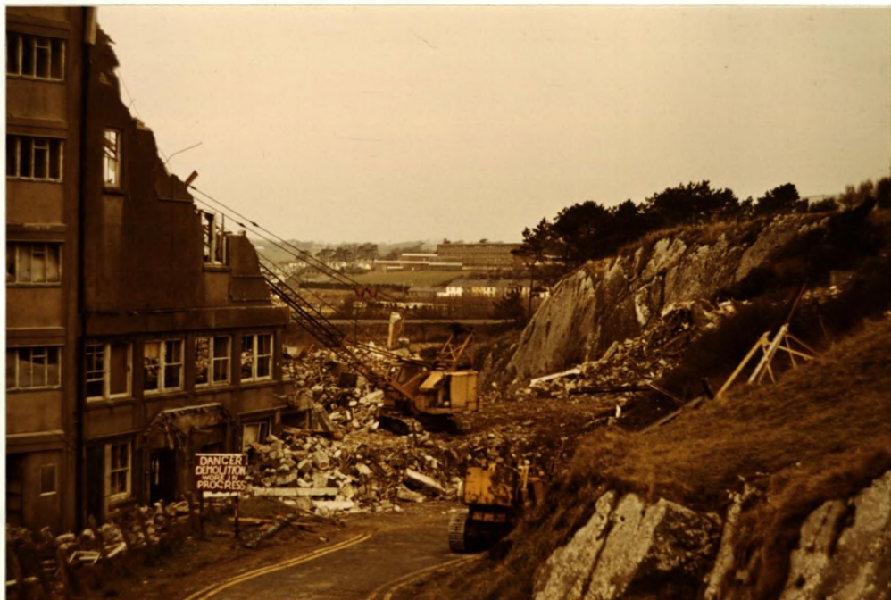
Fig. 2.15. Demolition of the 'Fundrome'.
