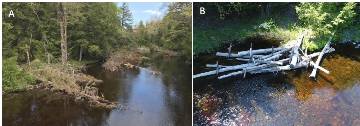
Figure 2-1. Examples of griphoist trees ("GH", A) and post-assisted log structures ("PALS", B) from the Narraguagus River
