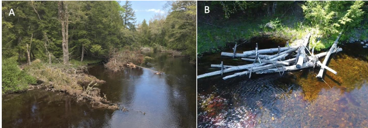
Figure 1-1. Examples of griphoist trees ("GH", A) and a post-assisted log structure ("PALS", B)
