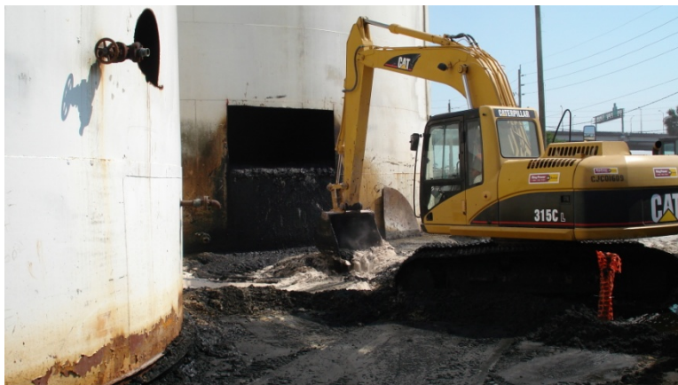
Figure 6. Removal and treatment of sludge in large tank
