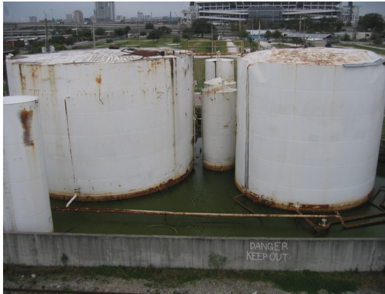
Figure 2. Tanks inside secondary containment system prior to 2008 removal action
