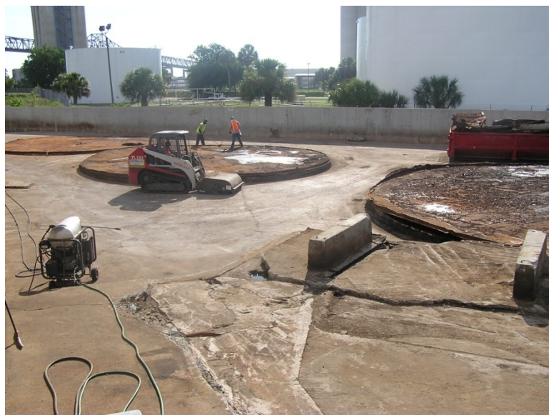
Figure 8. Final cleaning of secondary containment following demolition
