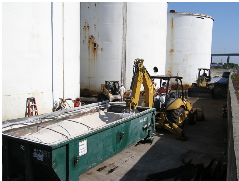
Figure 4. EZSORB ® solidification agent delivered to site in covered roll off box
