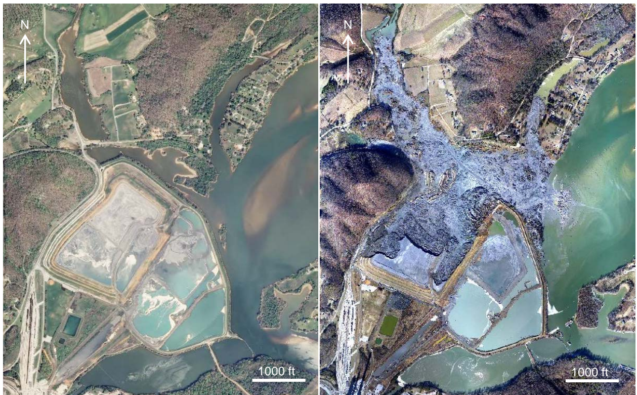
Figure 3. Comparison of aerial imagery before and after the 2008 failure.
