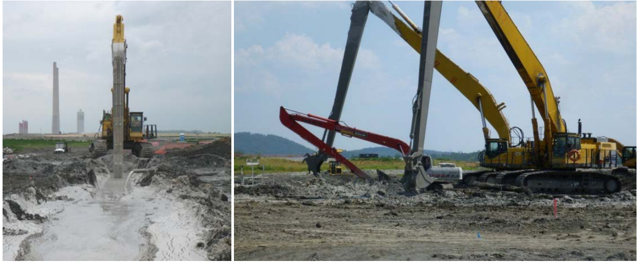
Figure 9. Slurry wall construction for the stabilized perimeter.
