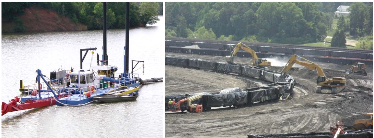
Figure 4. Dredging and load-out to railcars during Time-Critical ash removal.
