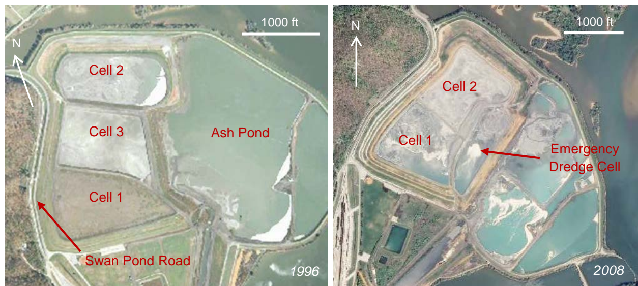
Figure 2. Aerial imagery of the ash pond facilities in 1996 and 2008.
