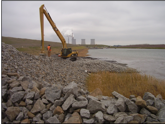
East Pond South Slope Buttress - Before
