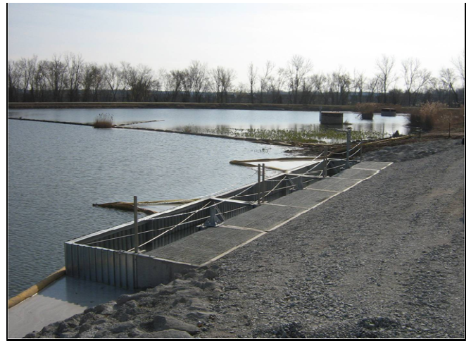
South Spillway Inlets - After
