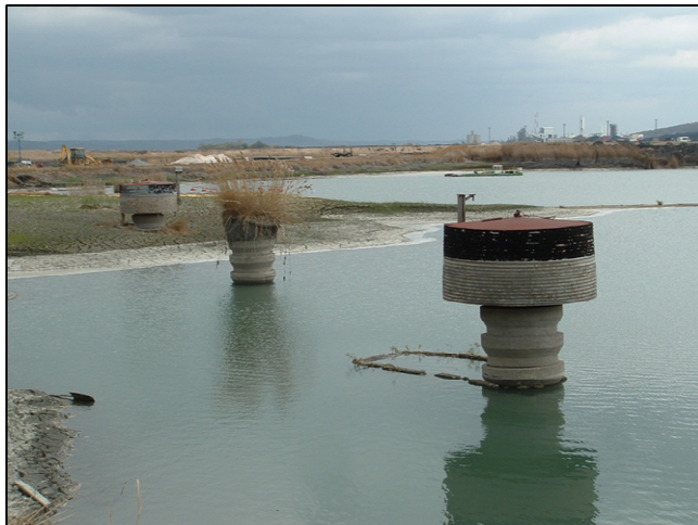
South Spillway Inlets - Before
