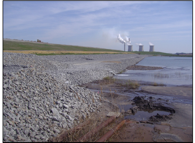
East Pond South Slope Buttress - After
