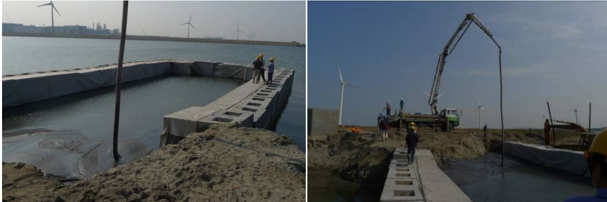
Figure 11 Photos of construction site
