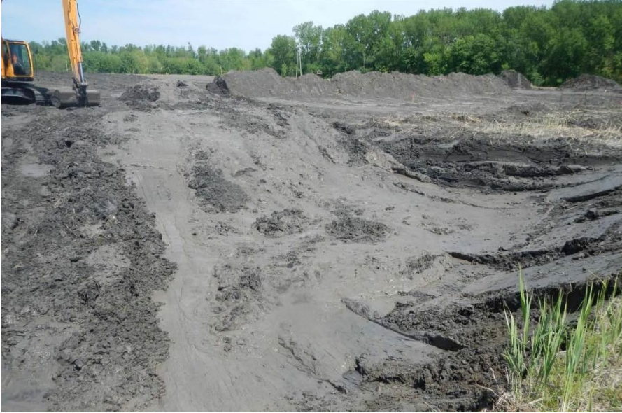
Figure 4: Saturated CCR at one edge of an ash pond.
