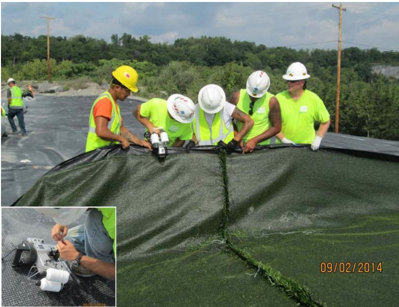
Figure 7: Geotextile component seaming using the sewing method.
