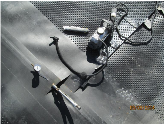
Figure 5: Air channel testing of geomembrane.
