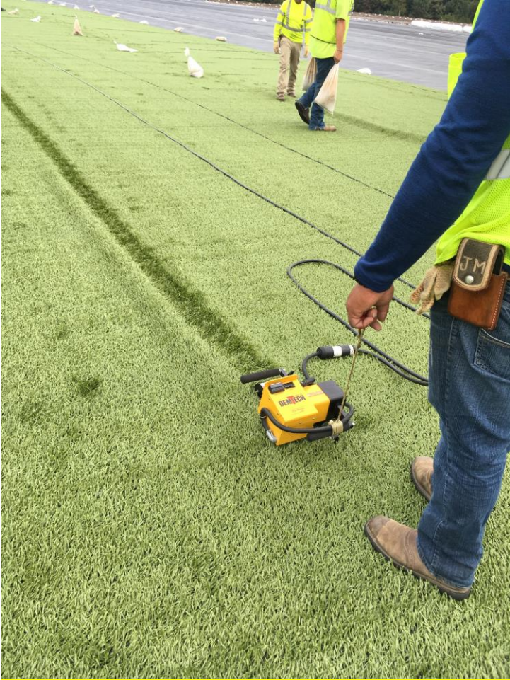
Figure 8: Geotextile component seaming using the welding method.
