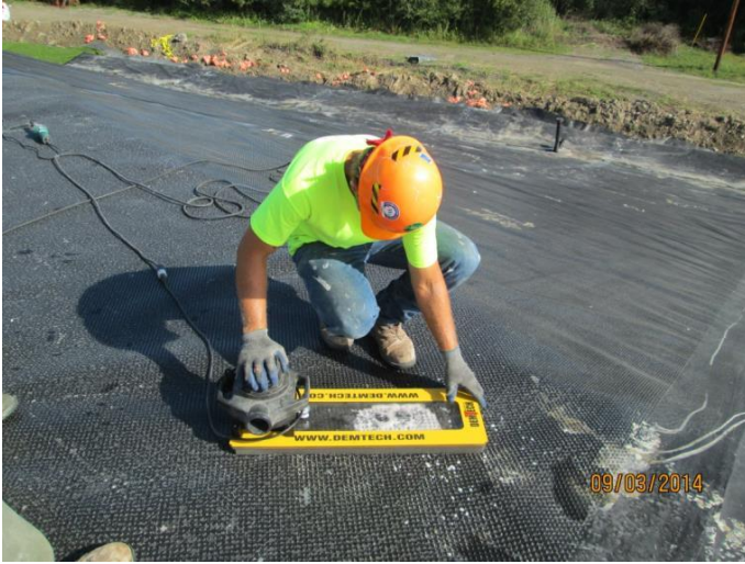
Figure 6: Vacuum box testing of geomembrane.
