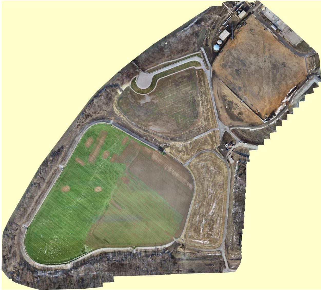
Figure 3: Ash ponds with ClosureTurf cap. Sand infill has begun.
