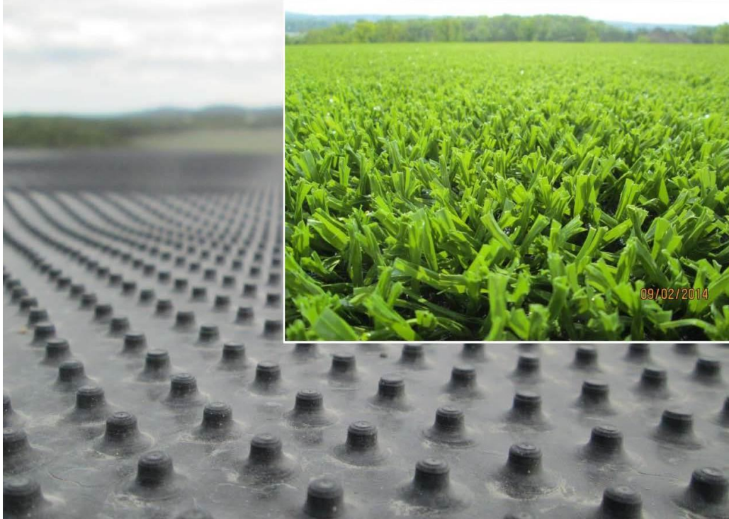
Figure 2: ClosureTurf ® cap installed components
