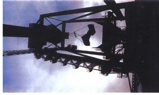
A clamshell grab coal unloading crane — Ashdod Port
