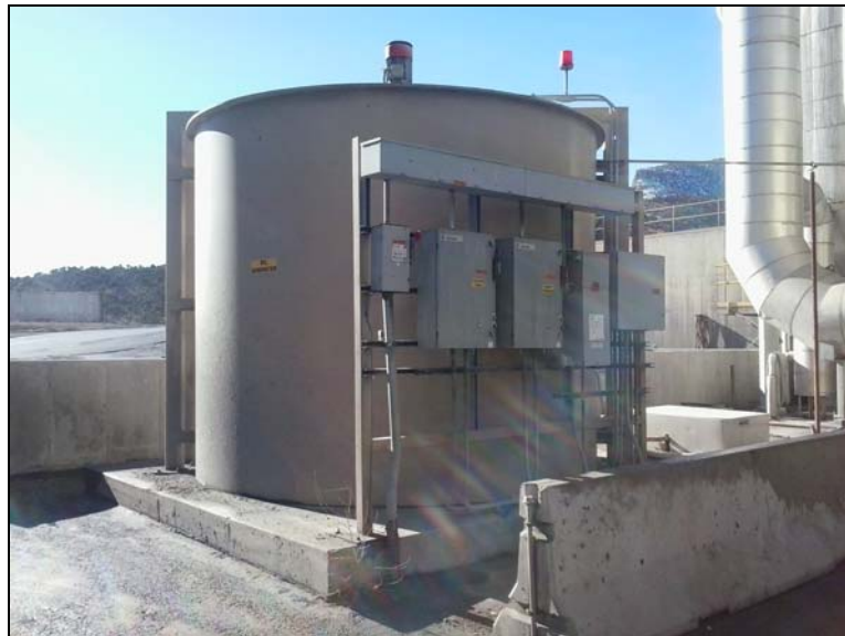
Figure 6 – RCC Concentrator Wastewater Tank
