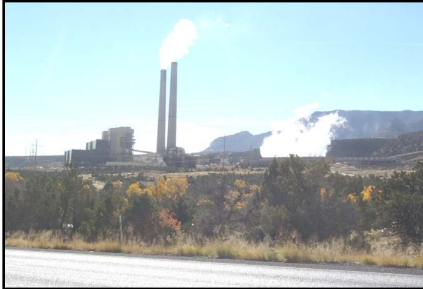
Figure 1 – Huntington Power Plant, Utah
