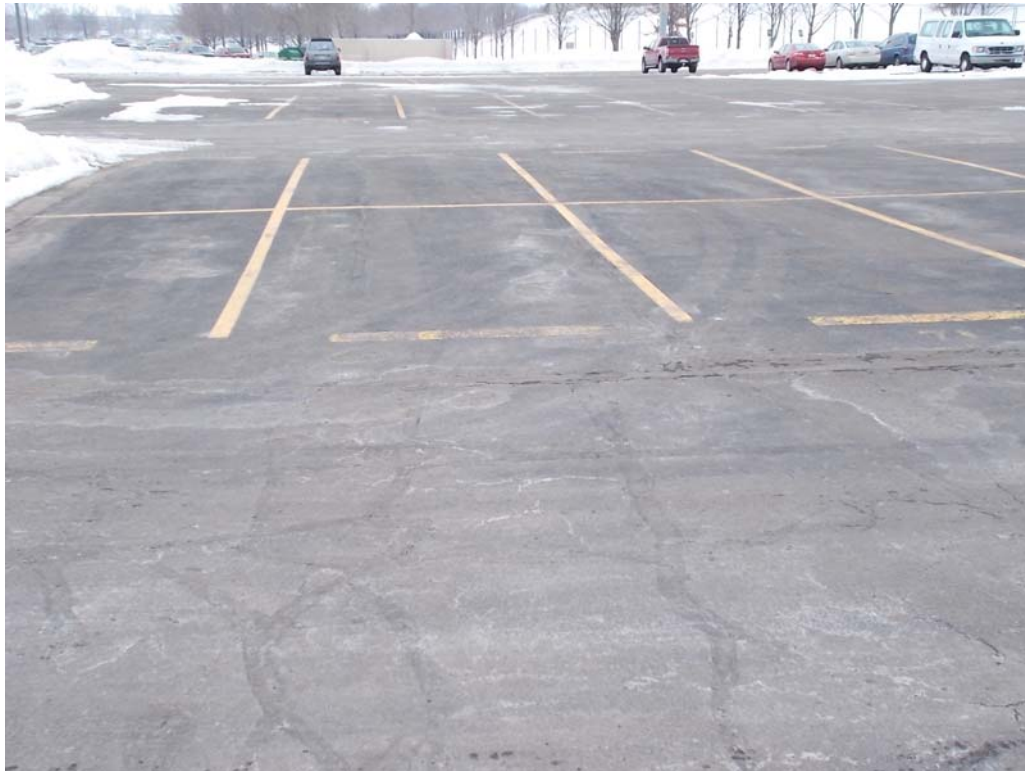
Figure 15. Stabilized parking lot section in November 25th of 2014
