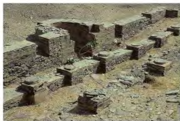
4-2 Ruined mosque, with remains of the qibla (wall facing Mecca), with a mihrab , and columns Soninke architects, c. AD 900 – 1500 (c. 350 – 950 AH) Stone Kumbi Saleh, Mauritania 2010 Photo: https://www.flickr.com/photos/72664388@N00/4852994797
