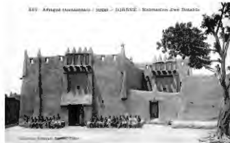
4-2 Potige (façade) of the home of an extended family Sorko architects, c. 1600 Adobe and wood Jenne (Djenne), Mali Undated postcard; c. 1910? https://en.wikipedia.org/wiki/Djenn%C3%A9#/media/File:Djenne_Fortier_407.jpg
