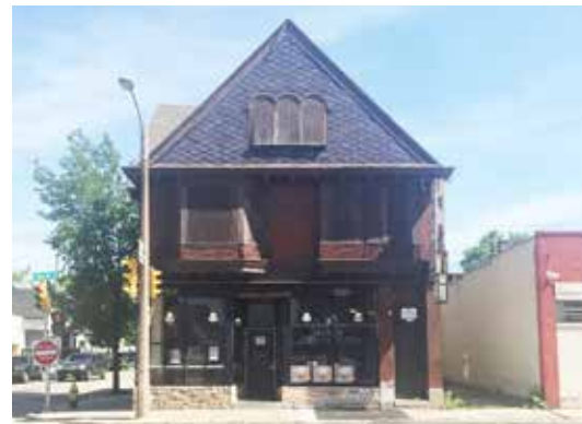
Jake's Deli existing facade
