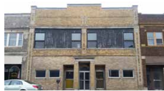
1511 Washington Ave existing facade
