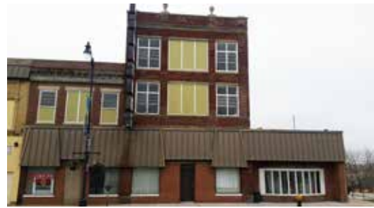
1322 Washington Ave existing facade
