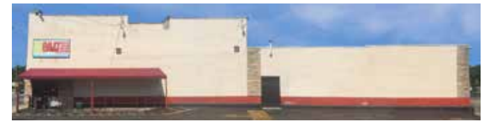
Galst Food existing East facade
