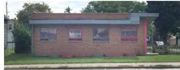
Existing Western facade
