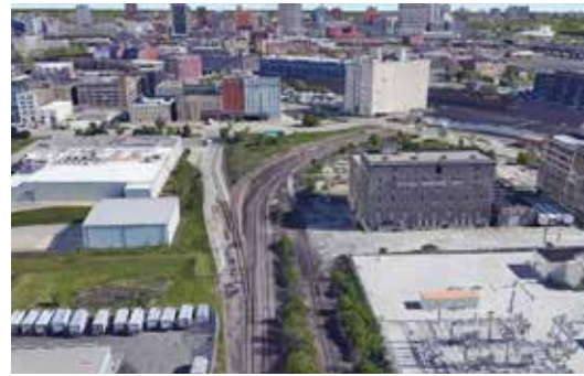
Existing - abandoned rails aerial
