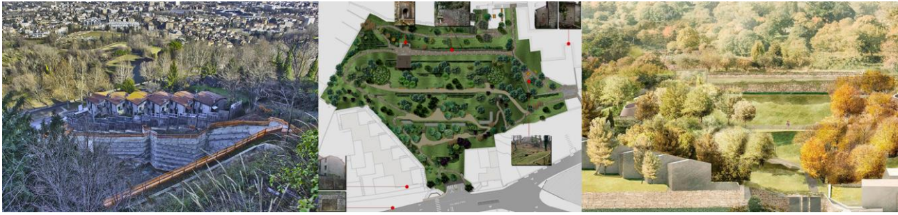
Figure 10. The construction site of the new parking in via Fara.
