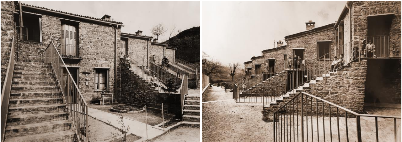
Figure 8. The Fanfani alla Fara houses after the construction in the 50s of the last century.
