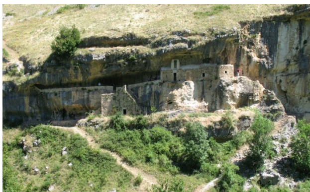
Figure 2. View from the valley in front of the hermitage
