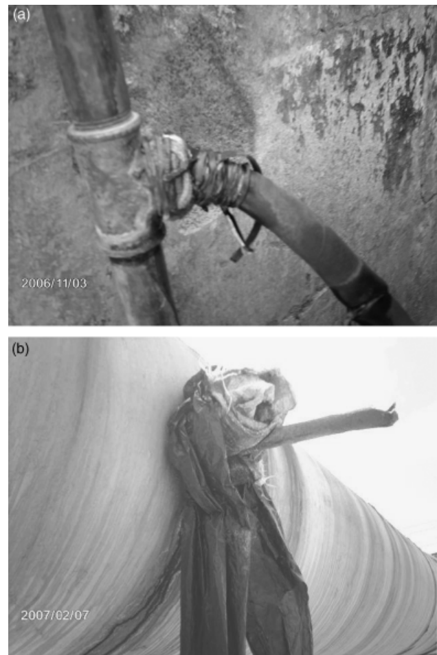
Figure 1 | (a) Illegal branch (Mfula 2007). (b) Draft inlet in Zambia (Chulu 2007).
