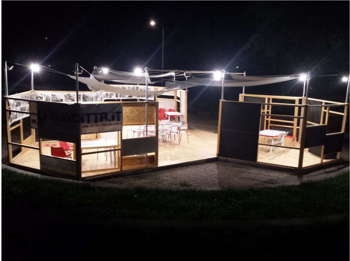
Figure 2. Night view of PAAI at Parco Savarino; the wooden structure is enriched by three different materials (one of each module): blackboard, which allows a temporary customization of the panels during the event, the mirrored film that allows a reflection in the space, and the metal sheet. The cover is made from a waterproof fabric.
