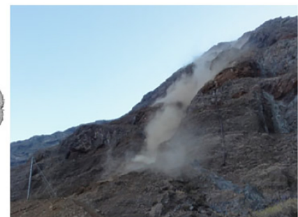
(a) Rockfall event over the Roquillos tunnel's northern entrance in El Golfo area
