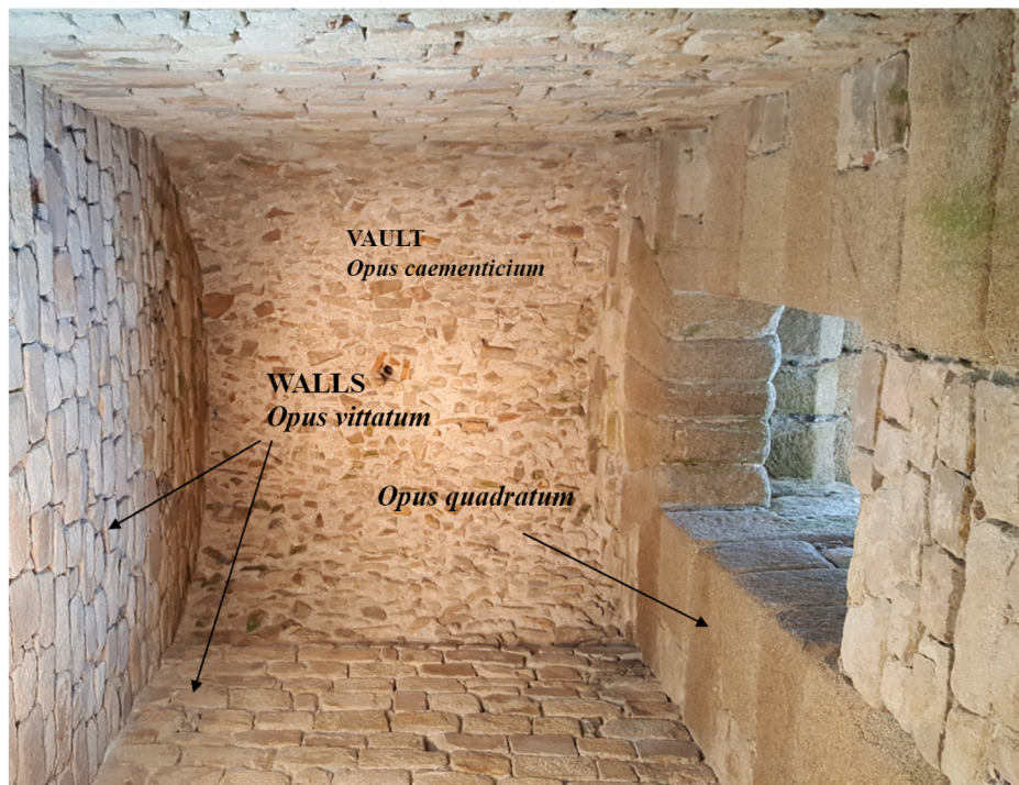
Fig. 3. Construction systems used in building structure.
